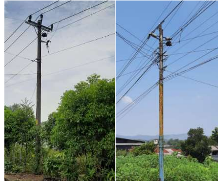
Gambar 4.15 Taping 1 Phasa 20 kV
