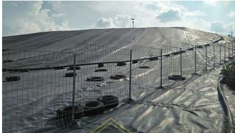
Gambar 2.7 Capping Geomembran PLTSa Jatibarang [25].
