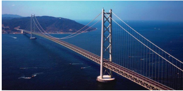
Gambar 1.1b. Jembatan Gantung (Suspension Bridge)
