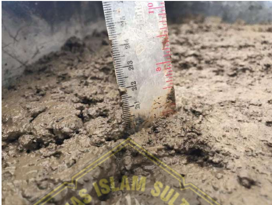
Pengukuran ketebalan base course
