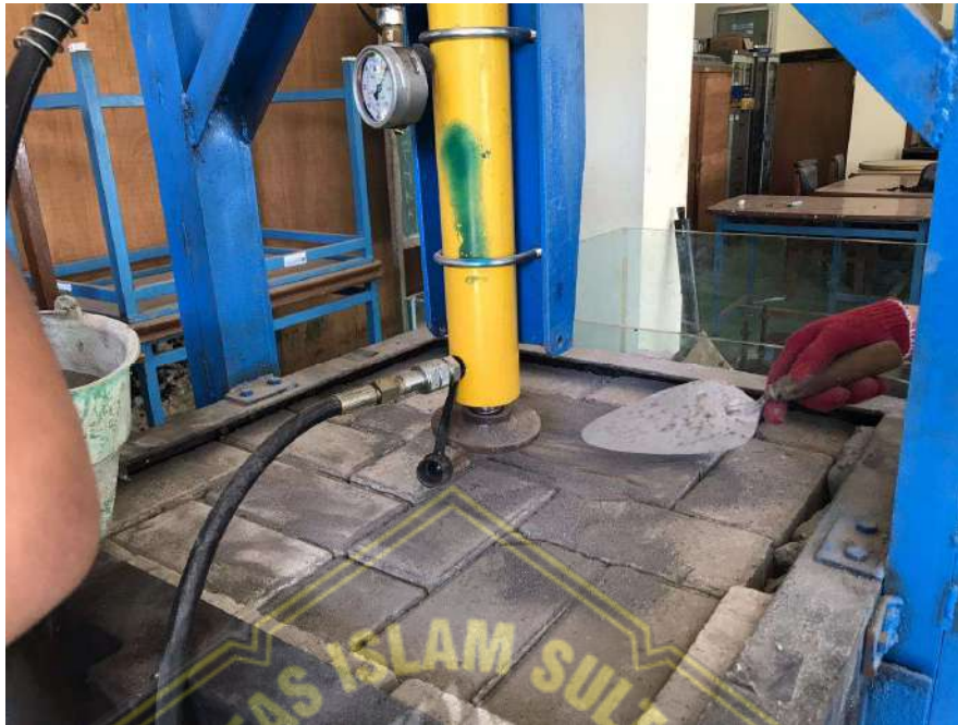
Pengisian jointing sand
