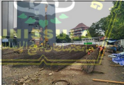
**Gambar 4.8 Fabrikasi Tiang Bore Pile**
