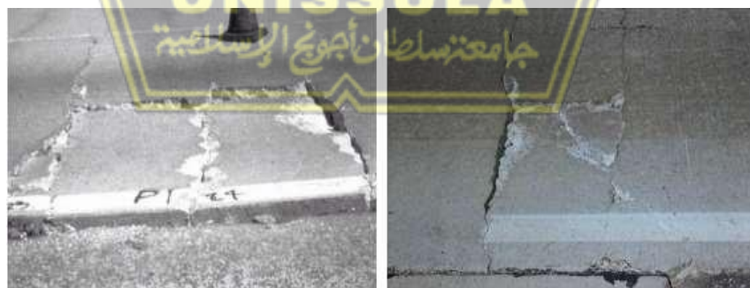
Figure 6.23. Examples of Punchout Distress
