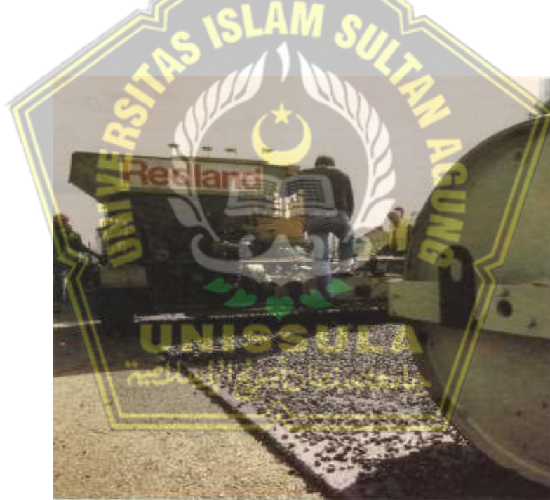
Figure 6.10. Photograph of Activity of Surface Dressing
