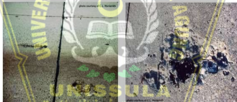
Figure 6.24. Examples of Popouts Distress
