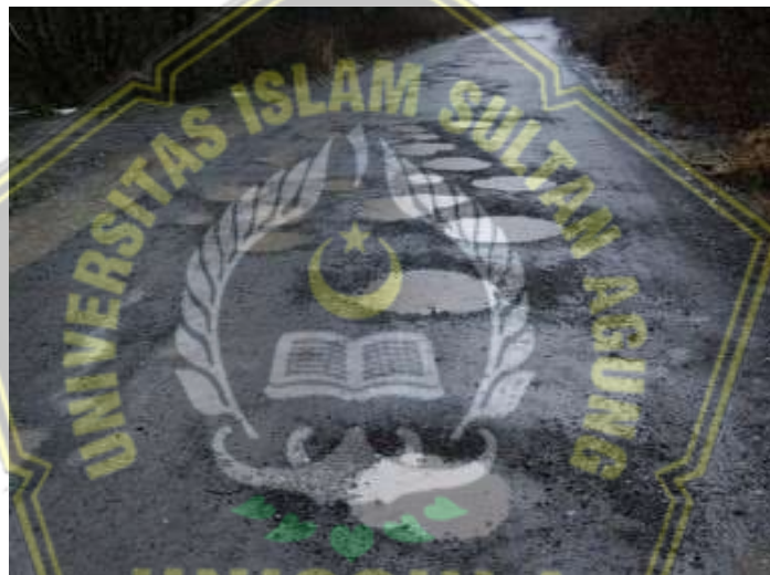
Figure 6.4. Potholes
