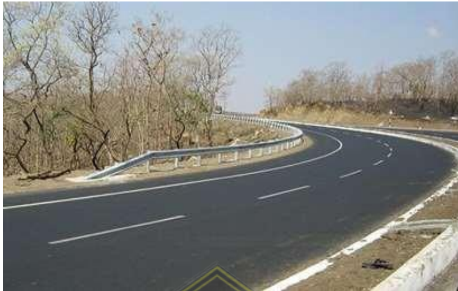
Figure 1.2a. Photograph of Flexible Pavement.
