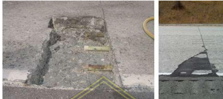
Figur 6.17. Example of a Dowel Bar Corrosion on the Left and on the Right a Patch Over an Area of Dowel Bar Failure
