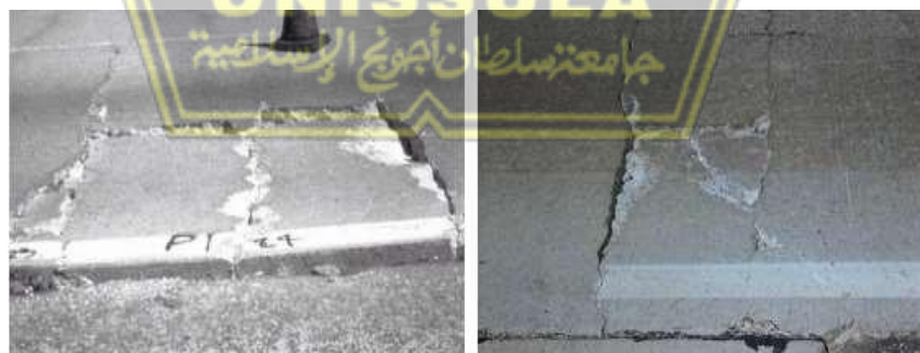
Figure 6.23. Examples of Punchout Distress
