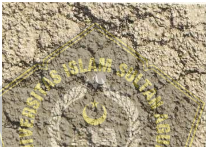
Figure 6.1. Crocodile crack occur in flexible pavement surface layer
