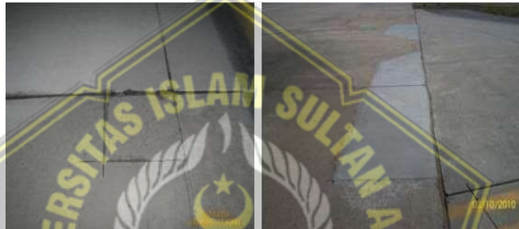
Figure 6.25. Examples of Slab Patching
