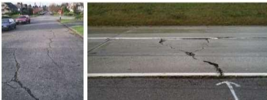
Figure 6.12. Examples of Longitudinal and Diagonal Cracks on the Left and on the Right Transverse and Diagonal Cracks [18]
