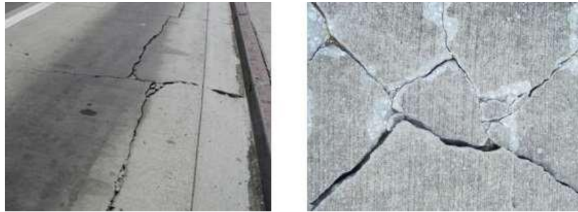
Figure 6.22. Examples of a Shattered Slab Distress [18]
