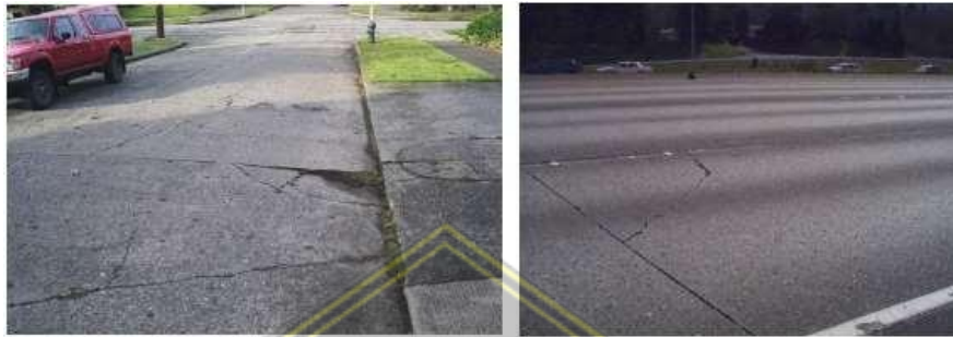
Figure 6.14. Examples of Corner Breaks at a High Volume Traffic Road
