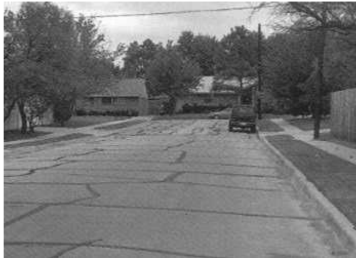
Figure 6. 7. Swelling in Flexible Pavement
