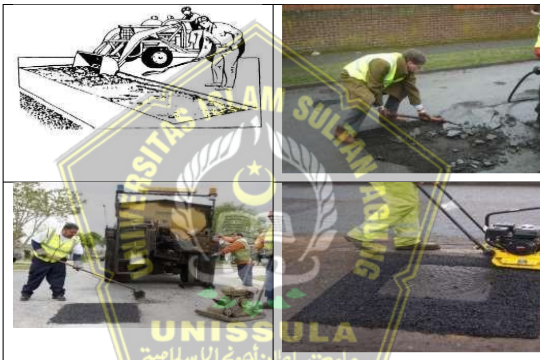
Figure 6.11. The Process of Repairing Cracks or Potholes on the Surface Pavement
