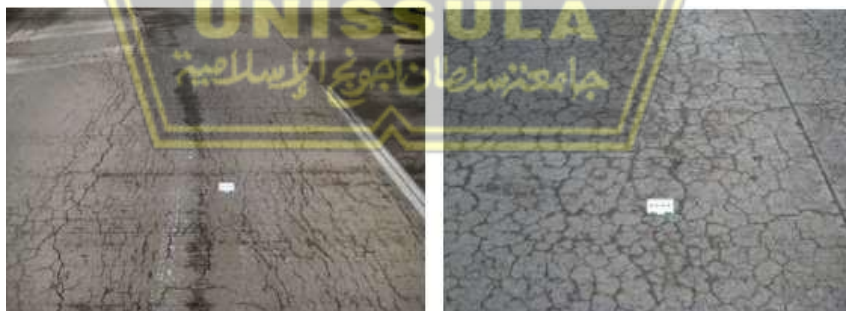
Figure 6.19. Examples of Map Cracking Resulting from Alkali-aggregate Reaction [18]
