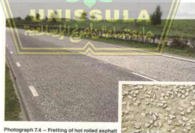
Figure 6.8. Raveling or Fretting in the Surface of Flexible Pavement
