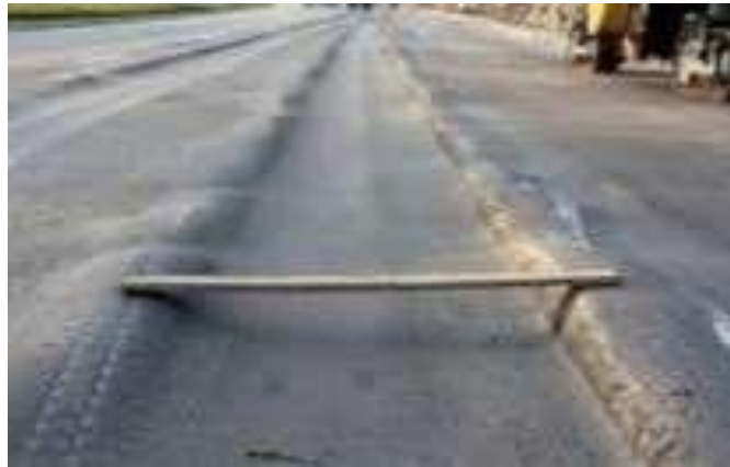
Figure 6. 5 Real-Time Formation of Ruts
