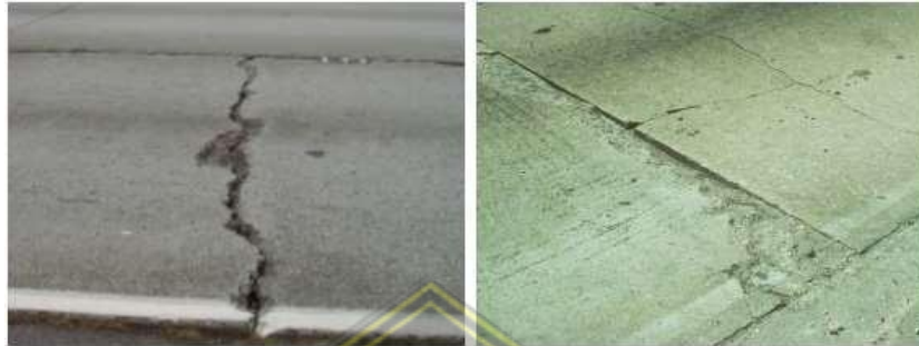
Figure 6.20. Examples of Spalling Along a Linear Crack on the Left and a Joint and Corner Spalling on the Right [18]
