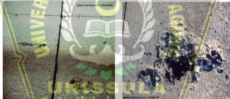
Figure 6.24. Examples of Popouts Distress
