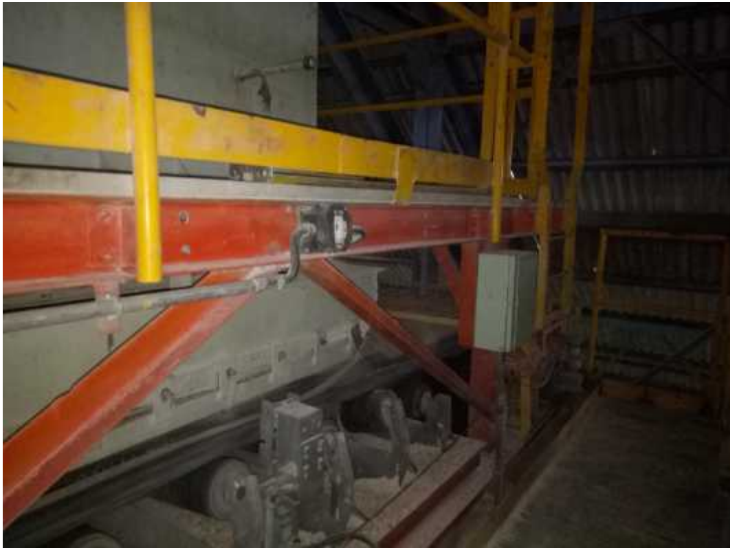
Gambar belt conveyor 244BC5
