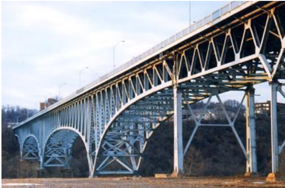
Gambar 1.5 Homestead Grays Bridge, Homestead - Pittsburgh's Greenfield district, Pittsburgh
