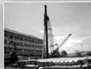
Piles Foundation for Building
