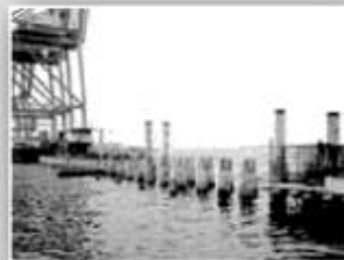
Piles for Marine Structure
