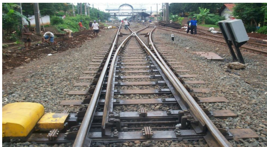
Figure 1.3. Railway switch
