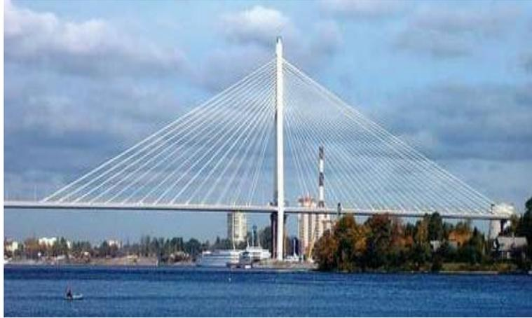
Gambar 1.4 Jembatan Cable Stayed (Sumber [4])
