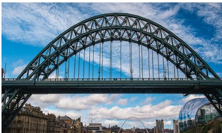
Gambar 1.3 Jembatan baja Through Arch (Sumber [3])
