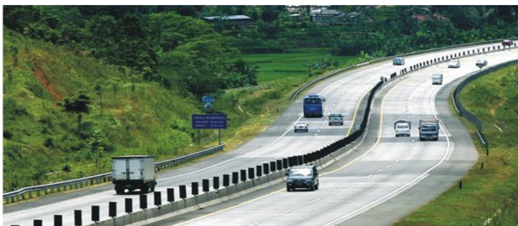
Figure 1.2. Typical existing toll road in Indonesia
