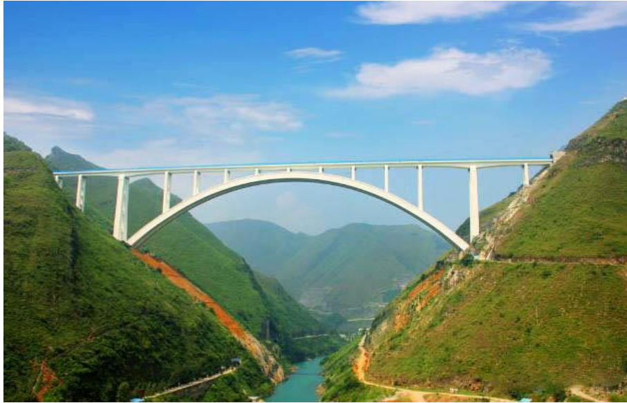
Figure 1. 2 Concrete Deck Arch Bridge (Source:[3])
