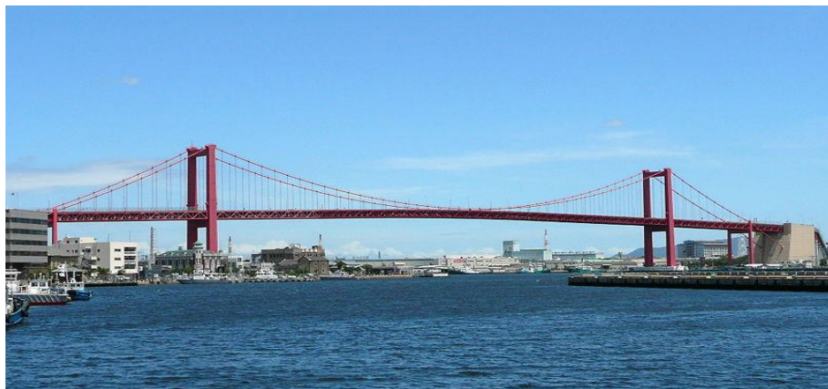
Figure 1. 5 Cable Stayed Bridge (Source:[3])
