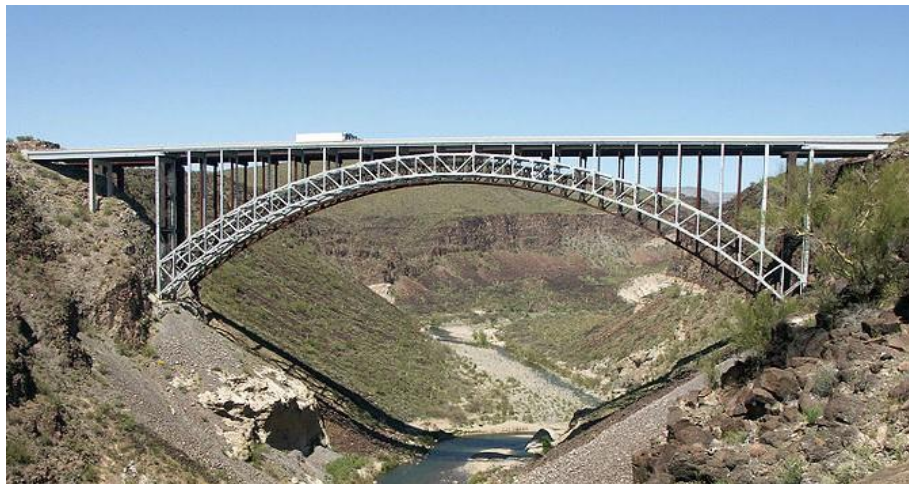
Figure 1. 3 Steel Deck Arch Bridge (Source:[3])
