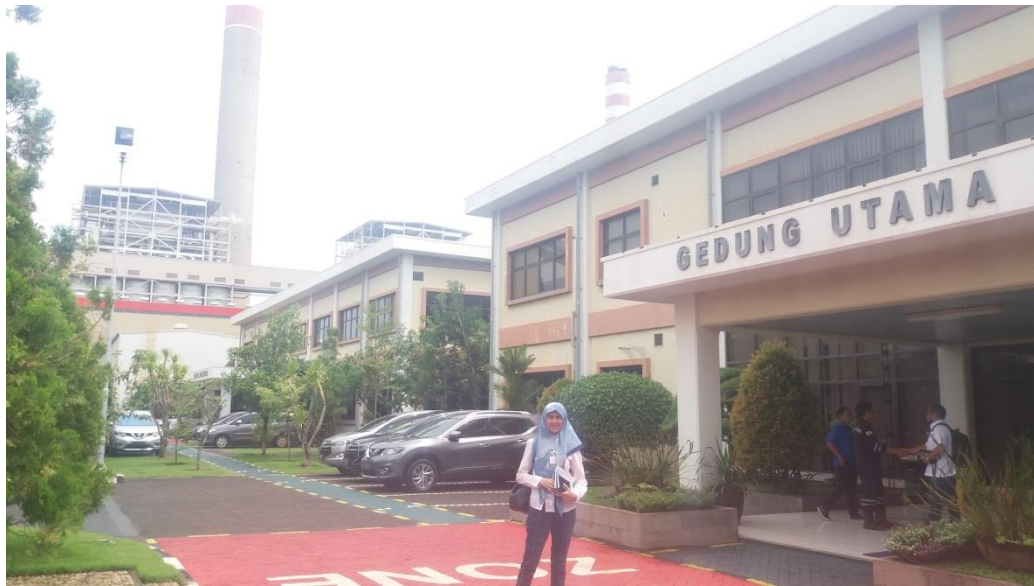
GEDUNG UTAMA PT. TJB POWER SERVICES
