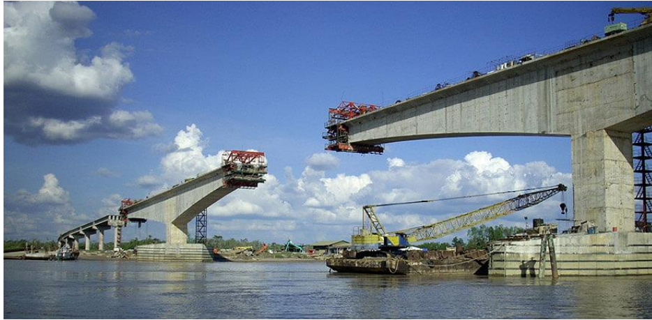
Figure 1.4 Cantilever Box Girder Bridge
