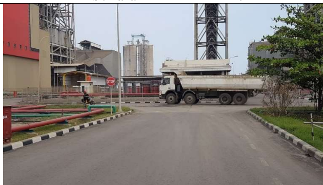
Pertigaan Hydrogen Plant
