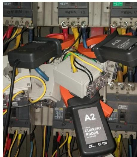
**Gambar 4. 11** Pemasangan Current Probe
