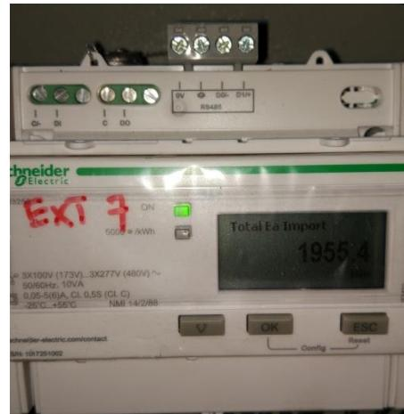
**Gambar 2. 5 Power Logic Schneider IEM 3255**
