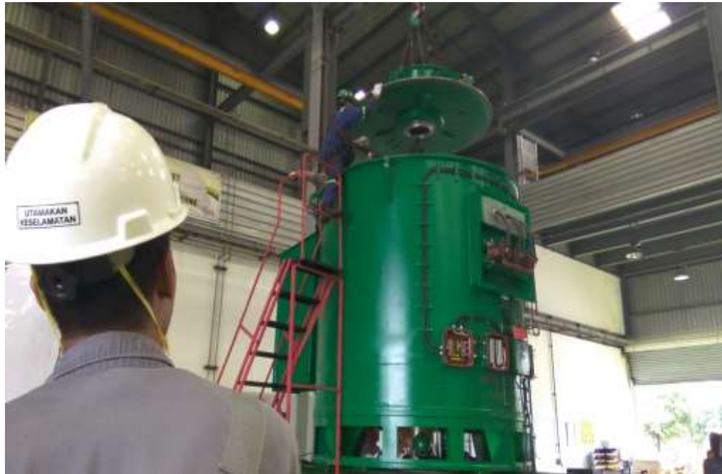
Lampiran 9. Pemasangan fan cover
