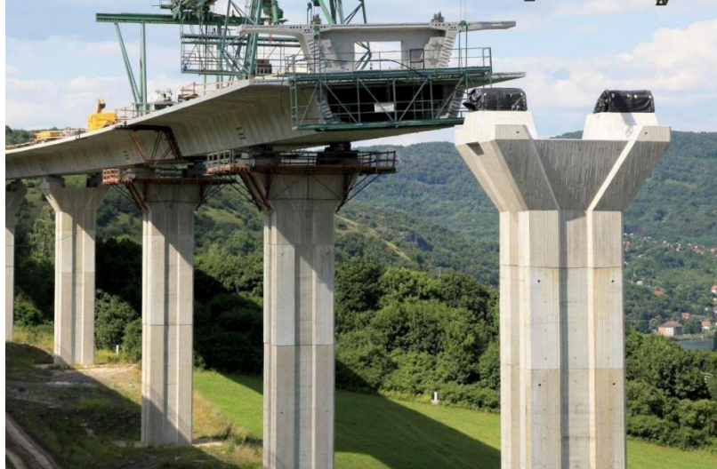
Figure 1.2. Bridge Box Girder under Construction
