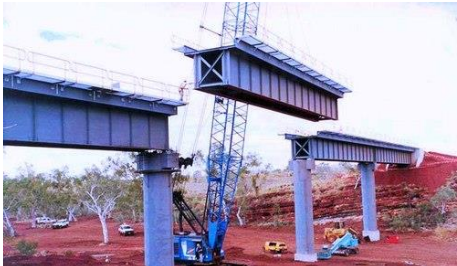
Figure 1.3. Steel box girder under construction
