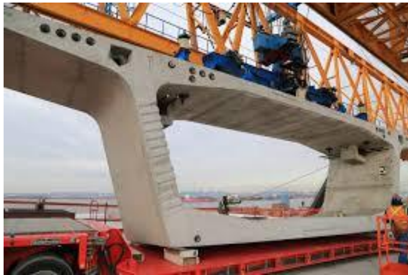
Figure 1.1. Pre-cast Concrete Box Girder
