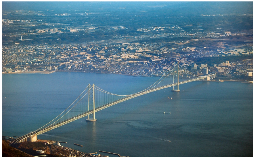
Figure 1.3. Suspension bridge, Akashi Kaikyō Bridge in Japan (Source [4])
