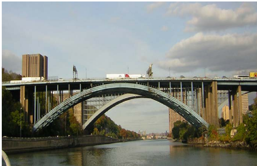
Figure 1.2. Alexander Hamilton Bridge, an open-spandrel arch bridge (Source [1])
