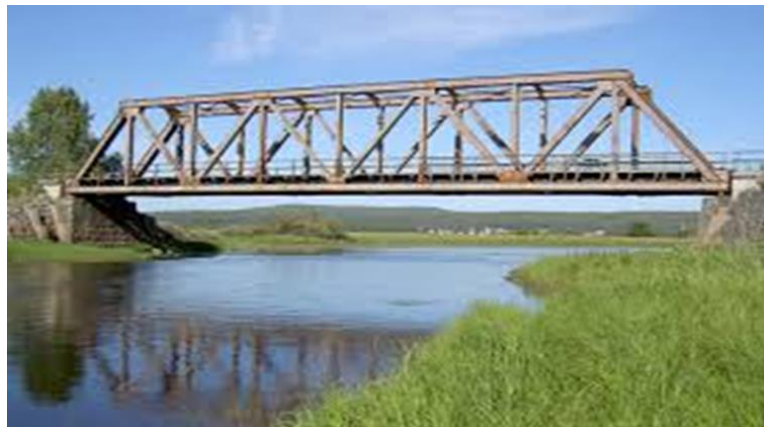
Figure 1.3. Steel-Truss bridge
