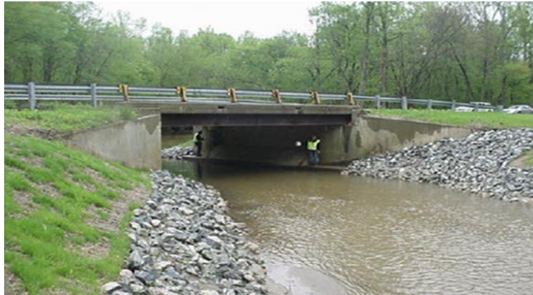
Figure 1.2. Simple Beam Bridge
