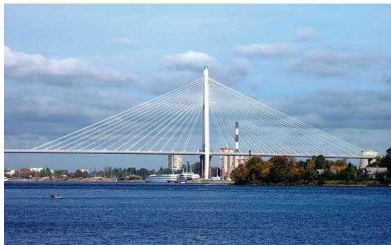
Figure 1.6. Cable-Stayed Bridge
