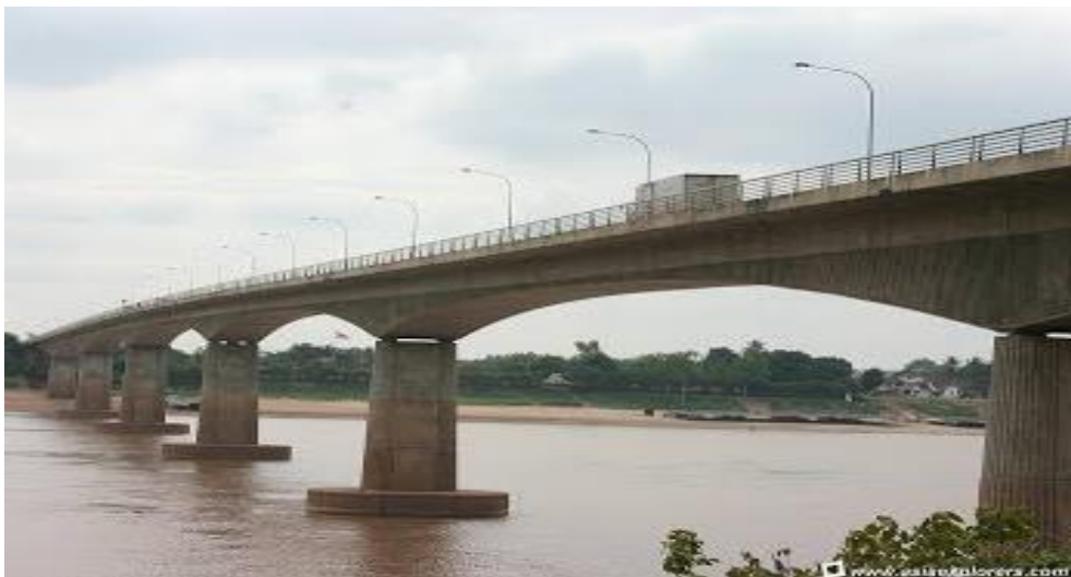
Figure 1.1. Bridge with some spans
