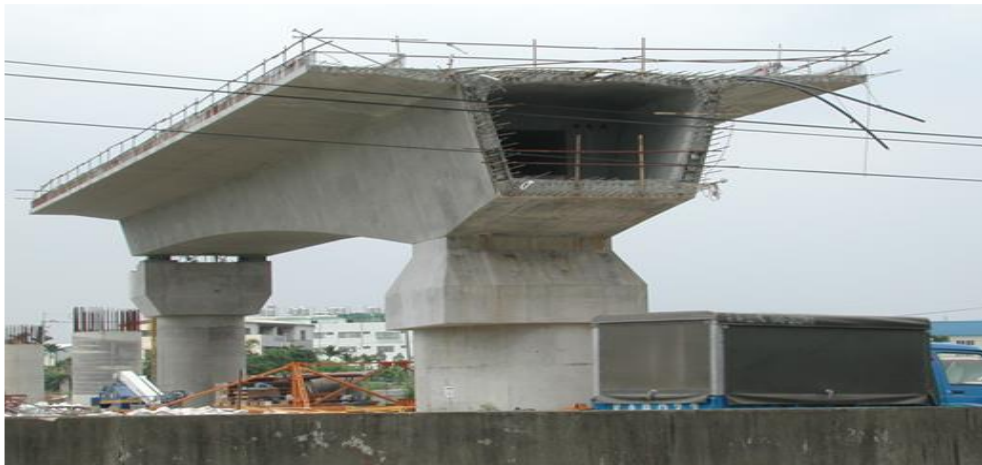
Figure 1.2. Types of Box Girder
