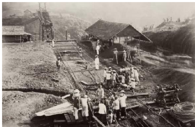
Figure 1.2 The construction of railway track in Java Island. Source [3]
