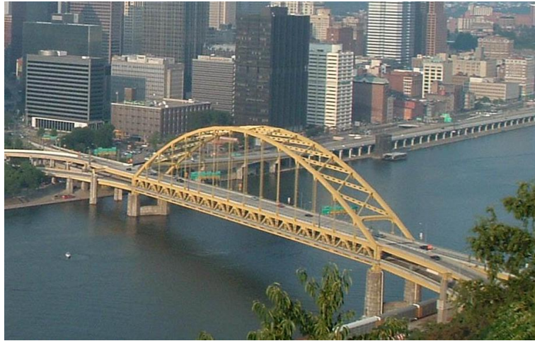
Figure 1.4. Tied arch bridge (Source:[6])
