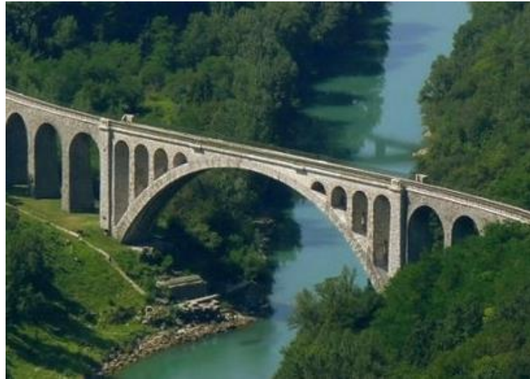
Figure 1.3. Arch bridge (Source:[5])
