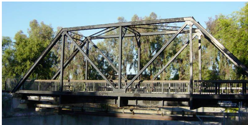
Figure 1.2. Truss Bridge (Source: [4])
