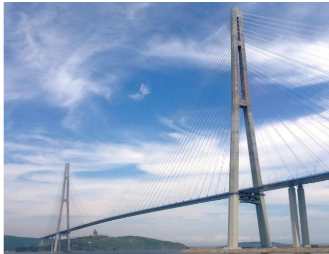
Figure 1.6. Cable-stayed bridge (Source:[9])
