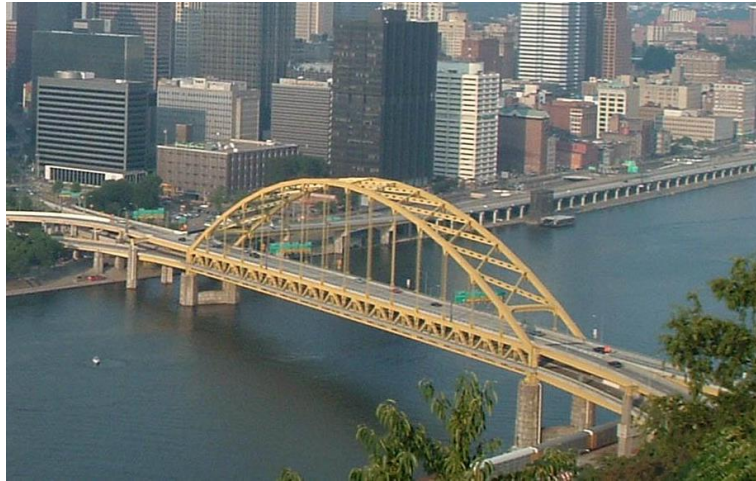
Figure 1.4. Tied arch bridge (Source:[6])
