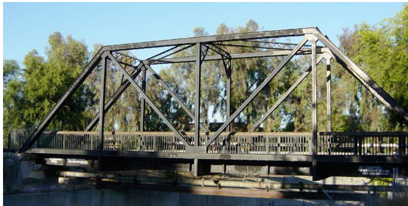
Figure 1.2. Truss Bridge (Source: [4])
