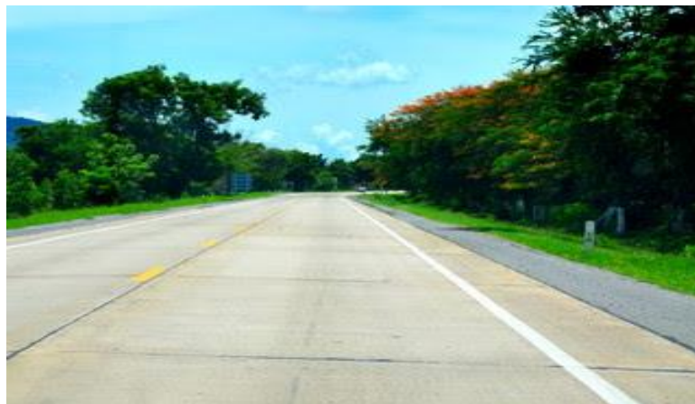
Figure 1.2b. Rigid pavement surface
